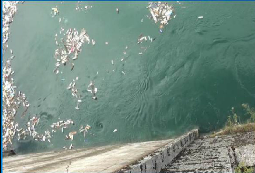
Vortex formation in front of the trash rack
