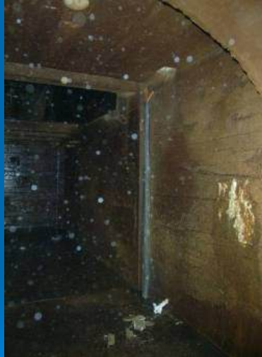
Installation of measurement equipment in turbine pit.
